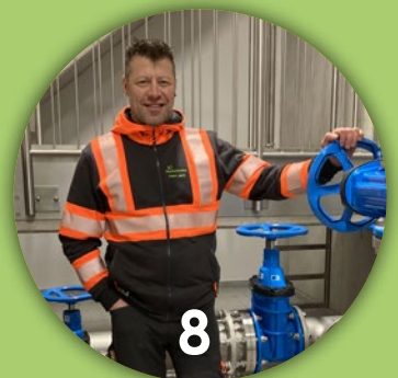
Neues Wasser- reservoir Hard
